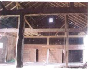
The beams in the barn are of similar construction, and the roof "trusses" consist of round logs, hand hewed on one side to support the roof boards. The outbuildings are very old, although their exact dates of construction remain uncertain.
